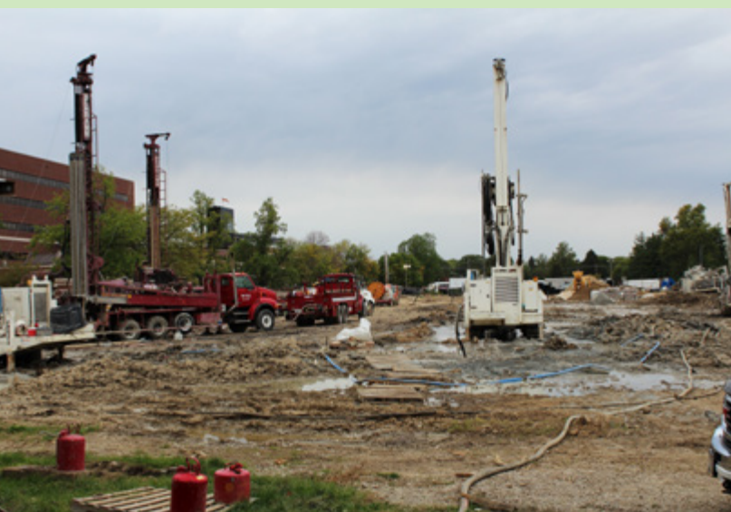
Figure 2: Geothermal borehole drilling. Photo by Lauren Jennings.
